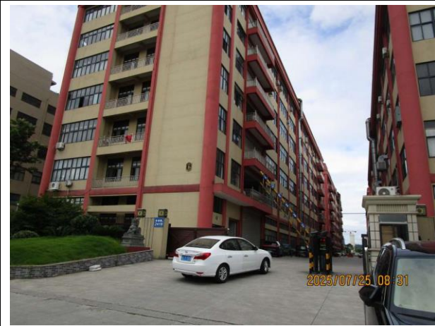
Auditee industrial gate gate
