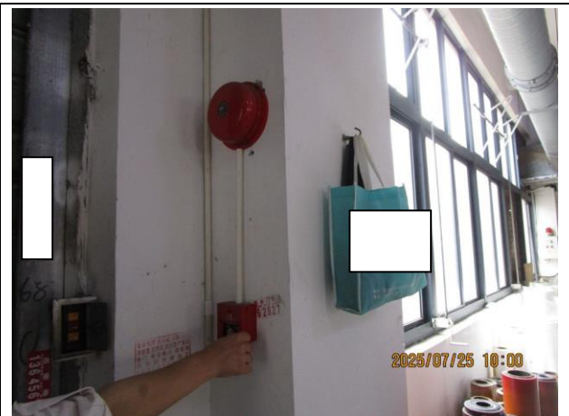
Fire alarm test
